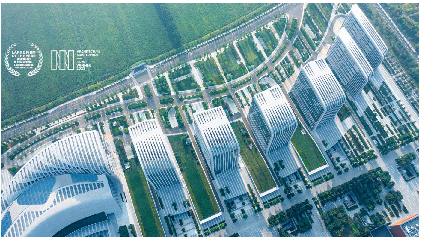
Jining Cultural Center, Jining, China
