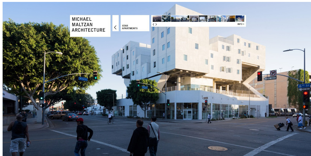
Michael Maltzan Architecture - LOCATION / Los Angeles, California TYPE / Affordable Housing, Social Services Counseling, Community Activities, Market-Rate Retail
